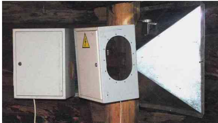
Figure 6 – Microwave treatment of the structure infected by borers
