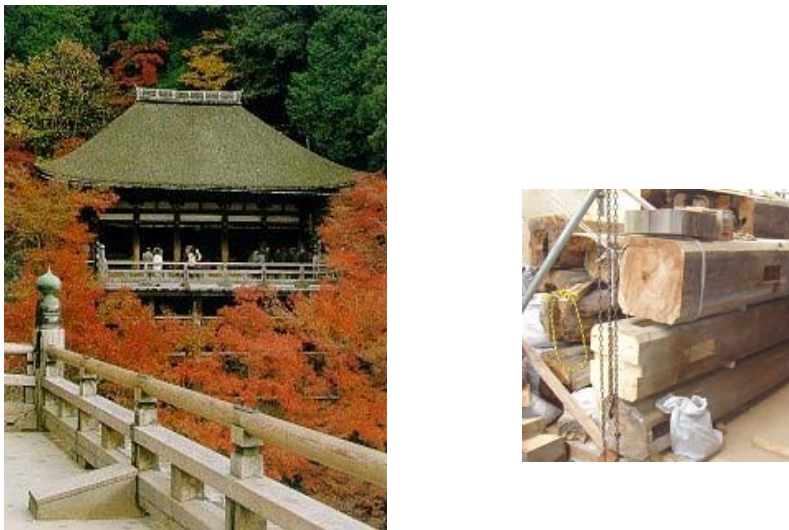
Fig.8 Okuno-in of Kiyomizu temple, Kyoto, Japan and some hozonzai , preserved wooden materials for a future reconstruction of the next generations at Kiyomizu temple.
